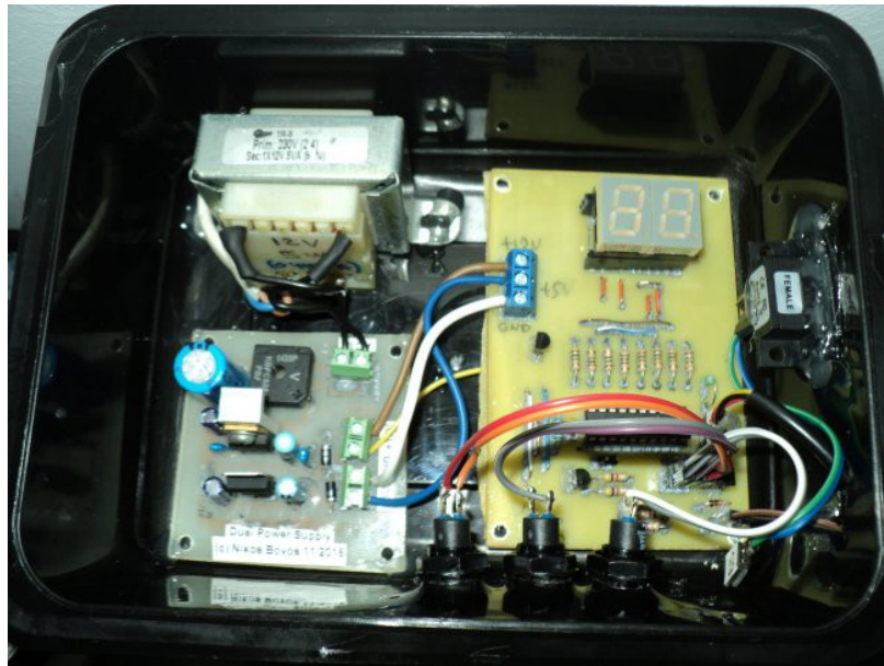
The final “box” of the project during installation
